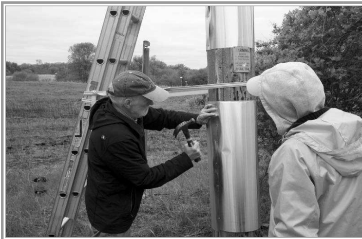
Julian Sellers nails a metal predator guard to an unused utility pole overlooking Benson Prairie. (Photo by Clay Christensen)
